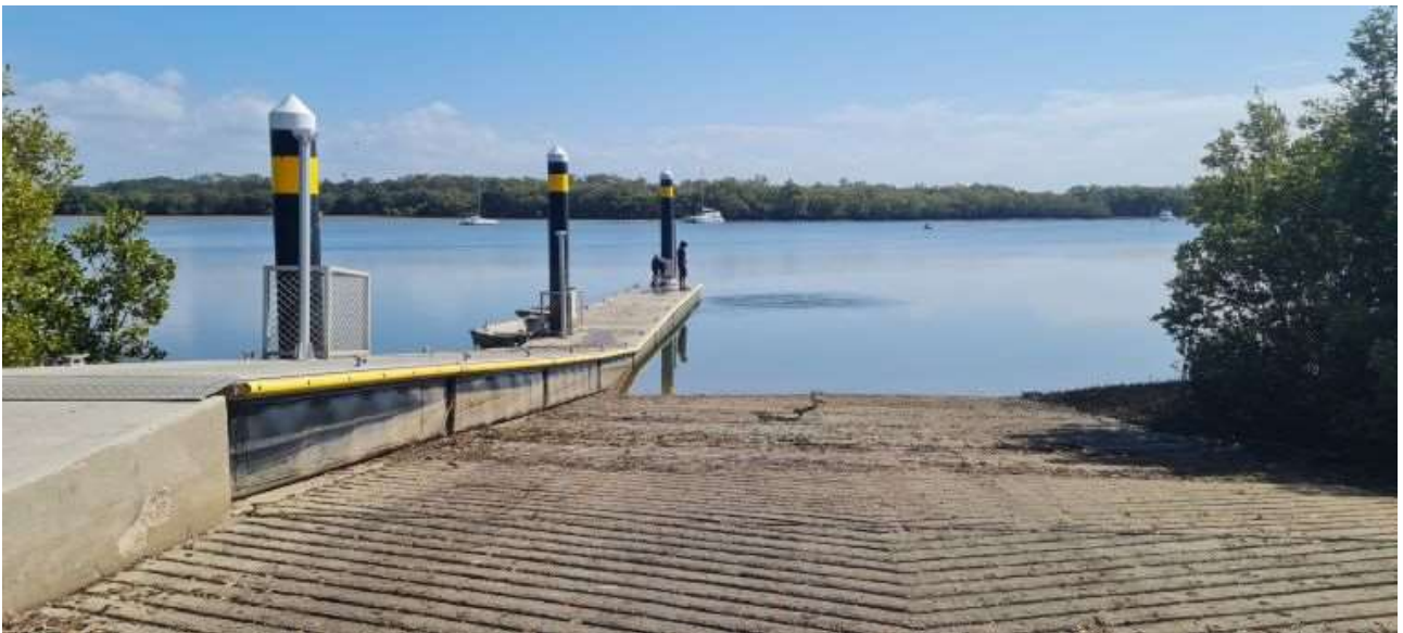
Photograph 8: This photograph was taken in August 2021 showing Location I.
