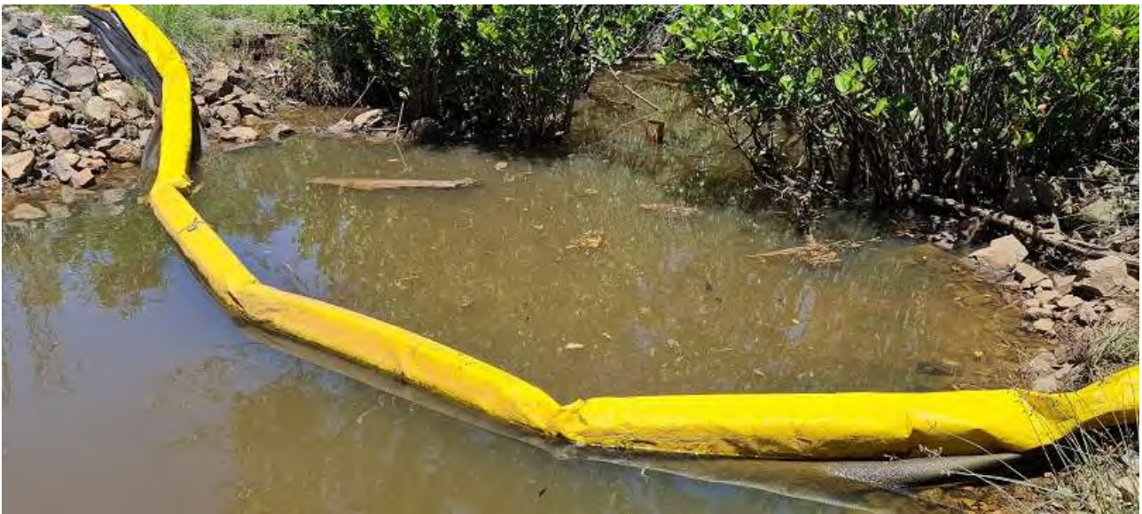
Photograph 4: Location D in December 2022 with sediment control boom installed downstream of the sample location.
