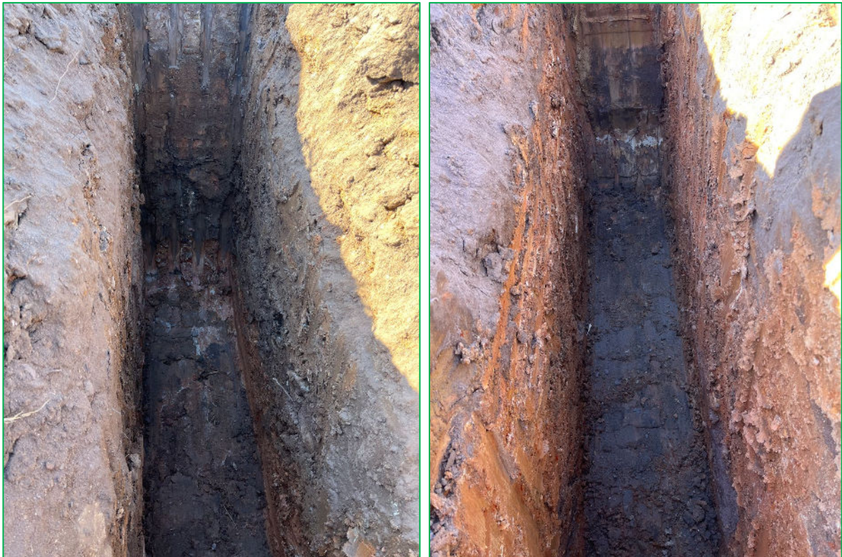
Figure 5: Typical Appearances of Test Pits Excavated Walls Across The Site
