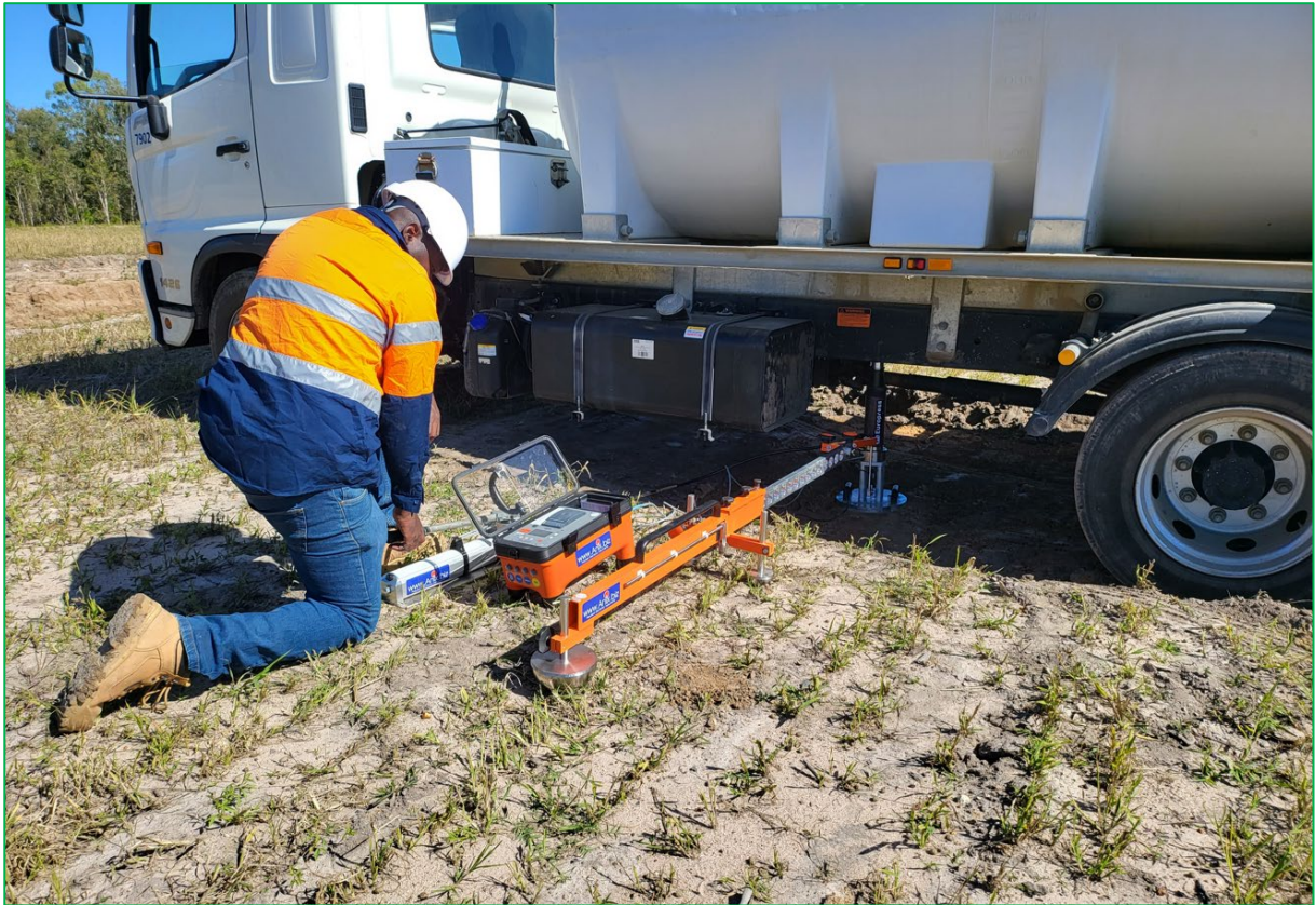
Figure 6: The Instrumented Plate Load Test Equipment Used for the Investigation
