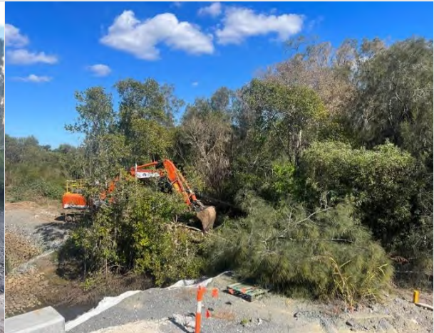
Figure 7. During Clearing Works
