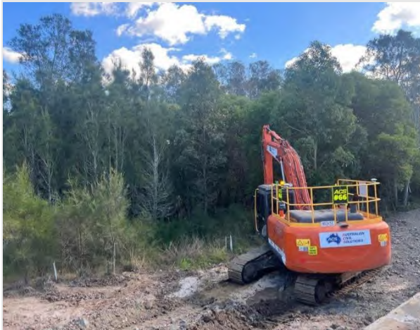
Figure 6. Prior to Clearing Works
