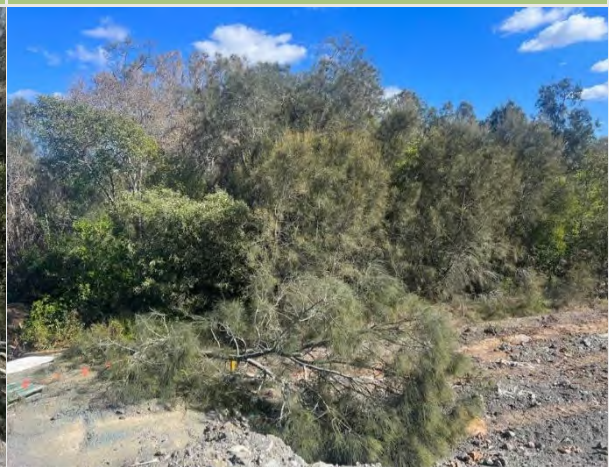
Figure 9. Post Clearing Works
