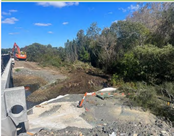
Figure 8. During Clearing Works
